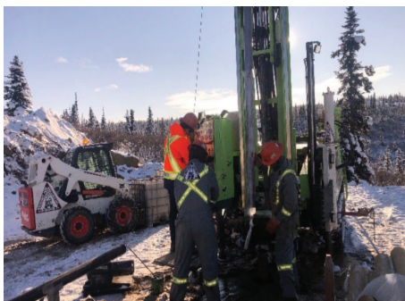
/ Geotechnical investigation drilling in the Secondary Heap Leach Facility footprint.
