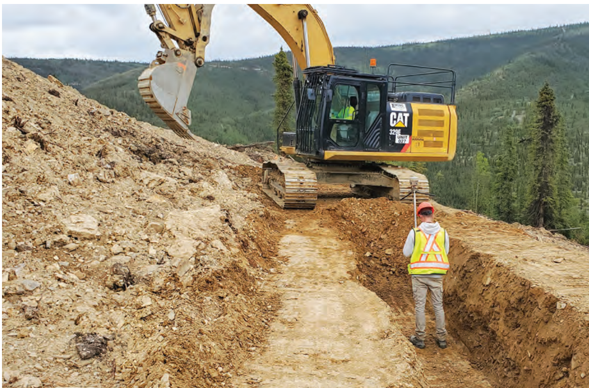
Underhill Geomatics Ltd. employee Niko Rodden surveying lateral ditches at Victoria Gold's Eagle Gold Mine.
