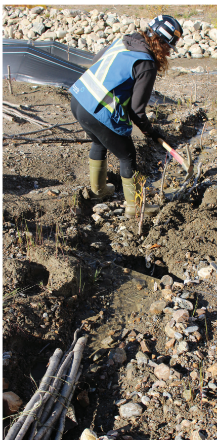
Willow staking and pole drain repair at the Eagle Gold Mine.
