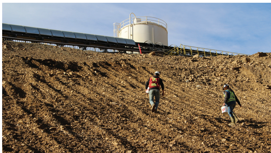
Seeding and willow staking during Victoria Gold's environmental program at the Eagle Gold Mine.
