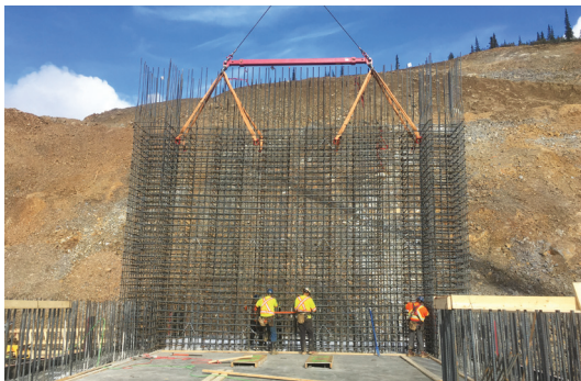
Yukoners at Work: Installing rebar at the Primary Crusher and preparing foundations at the Secondary Crusher, with the camp in the background.
