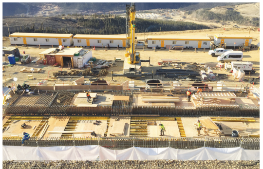
Yukoners at Work: Installing rebar at the Primary Crusher and preparing foundations at the Secondary Crusher, with the camp in the background.
